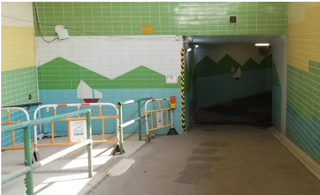
Photo 3 - Erection of site hoardings in unobtrusive colours
