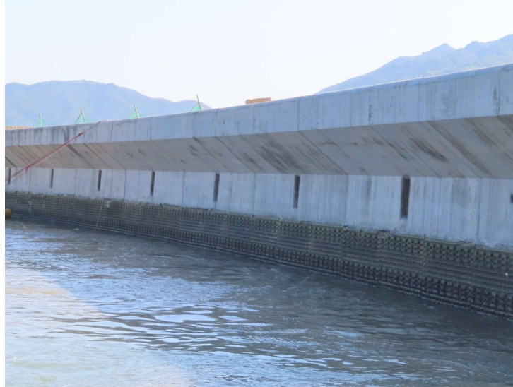
General View of Vertical Eco-shoreline
